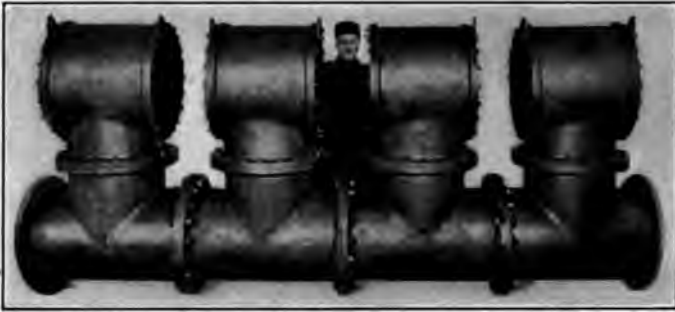
FIG. 238.—Smith tar extractor. Capacity 250,000 cu. ft. per hour.
